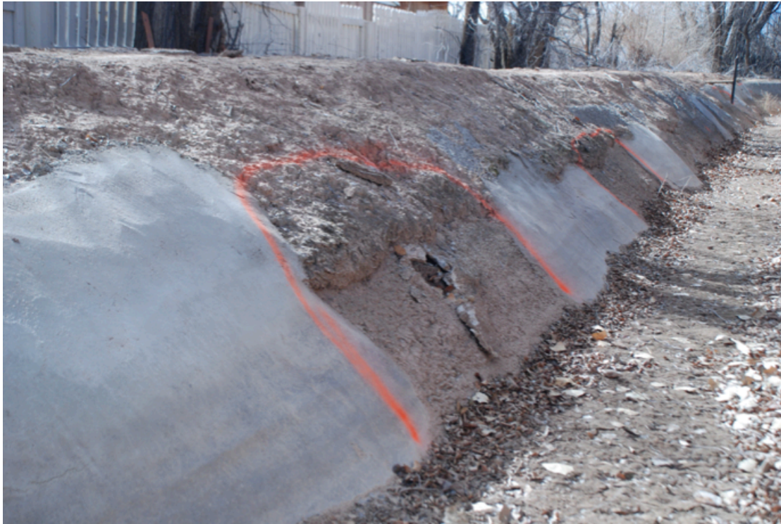
Sample of failure between patches, under more aggressive repair program areas between patches when a failure is discovered entire area between patches is replaced.
