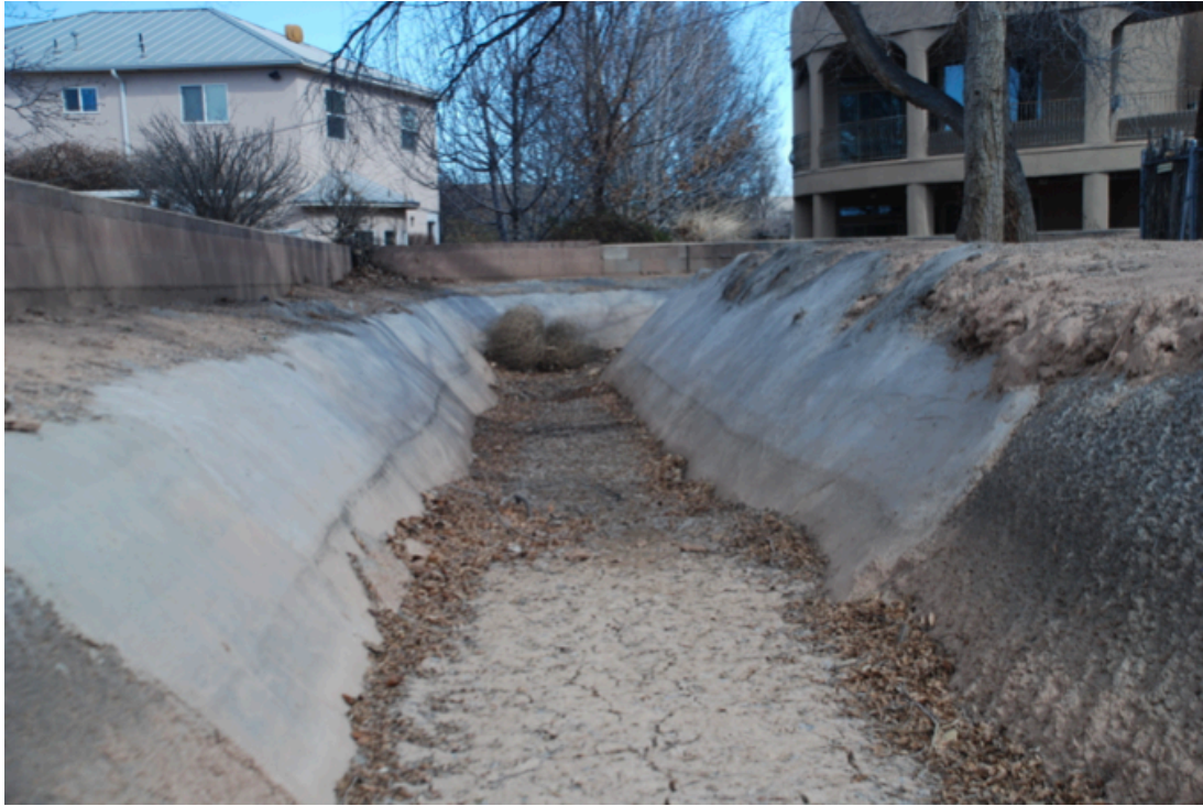
Example of a large repair replacing piecemeal patching
