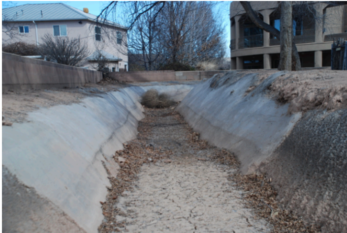
Repaired sidewall in foreground, original gunnite downstream
